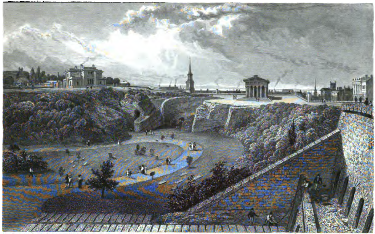
ST. JAMES'S PARK EMBANKMENT, LONDON, ENGLAND. LOOKING NORTH.
